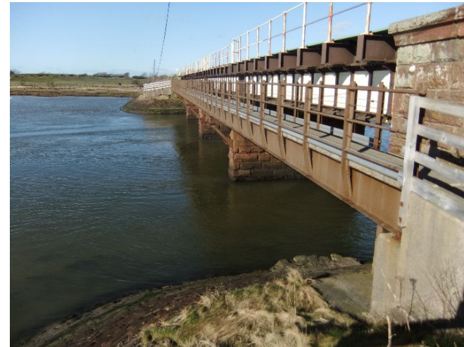
River Mite Viaduct with cantilevered crossing
