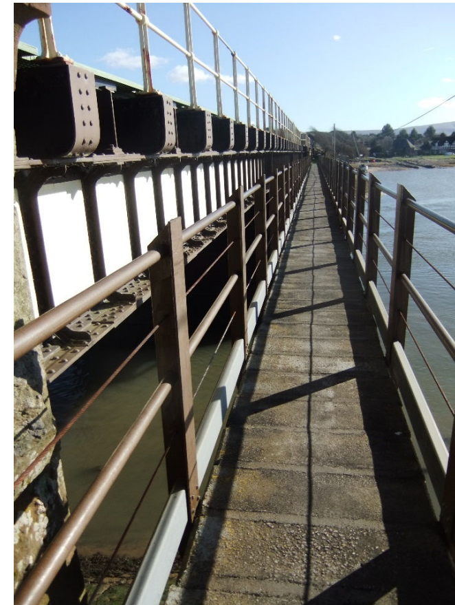
River Mite crossing – existing narrow walkway cantilevered off the railway viaduct
