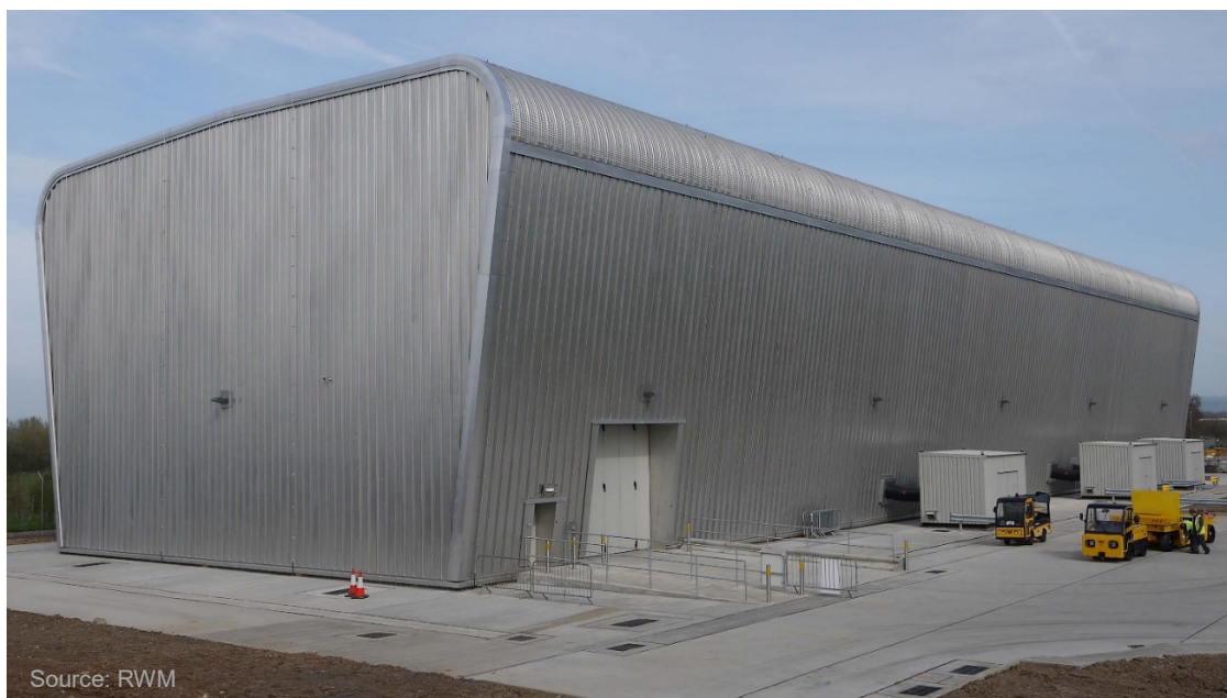
Figure 2. Interim storage facility
